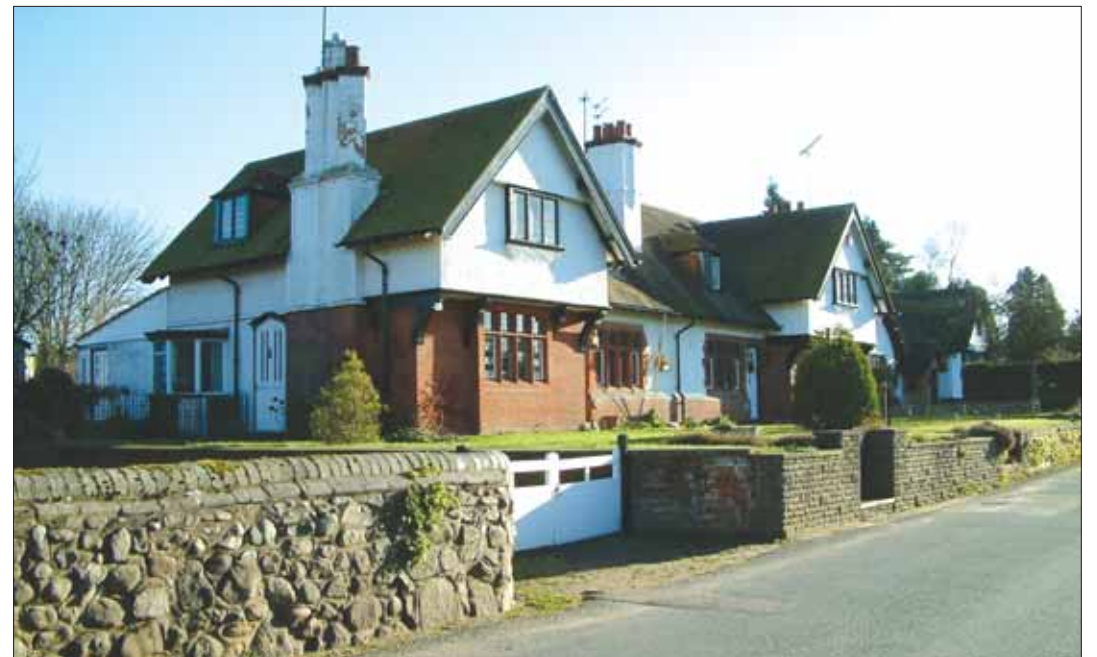
Alms house style cottages in The Holloway at Trysull which make a major contribution to the Conservation Area there.
