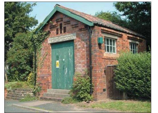
Electricity switch house
