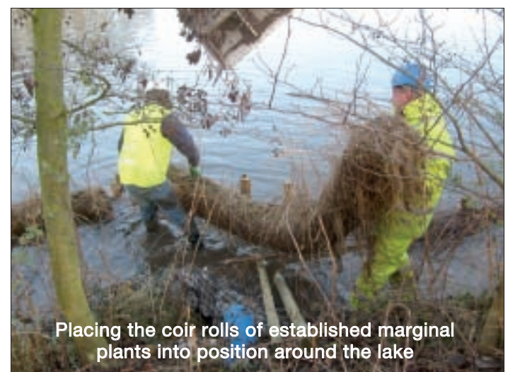
Waterside planting and edge stabilisation under construction
