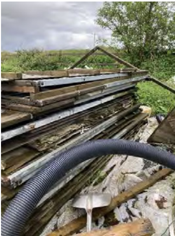
Fig. 1c – remaining sections of Previous Stables – dilapidated and unfit for re-use
