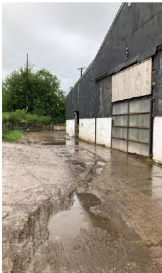
Fig. 3c – accessway to Stables past the Barn
