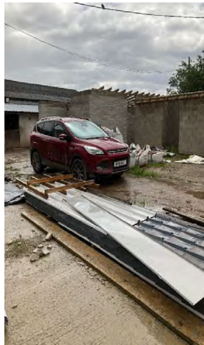
Fig. 4b – view to the southwest, taken within the courtyard
