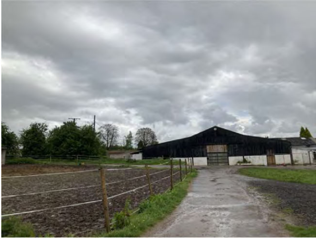
Fig. 3d – Stables located to the left hand side of the Barn, viewed from the manège
