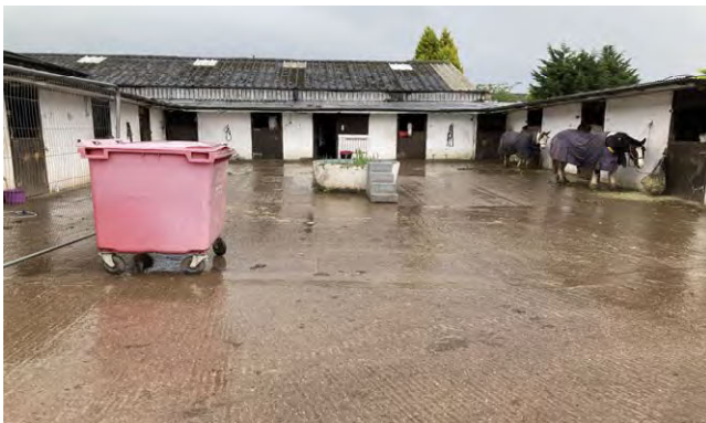
Fig. 2c - Courtyard Stabling – breeze block construction with corrugated roofing
