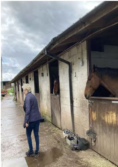
Fig. 2b - Additional Stables – breeze block construction with corrugated roofing
