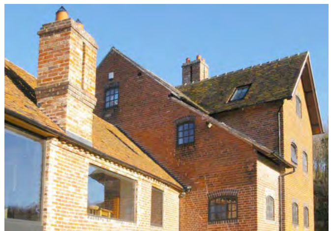
This barn conversion incorporates both modern and original features, with careful attention to maintaining a rhythm in the window openings, and retaining the hierarchy of scale between the original house and the later extensions.
