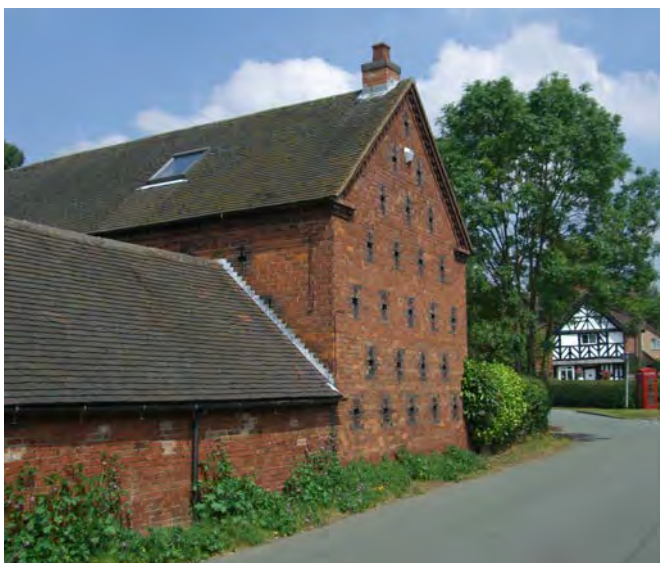
This successful barn conversion retains the original brick detailing whilst simple roof lights have been used to bring light into the building without compromising the traditional form.
