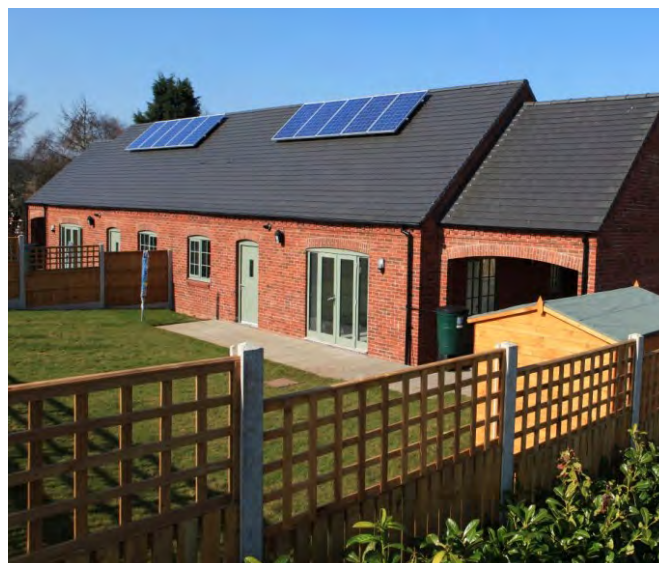
This development on Himley Lane, Swindon, uses the traditional farmstead layout - common in South Staffordshire - whilst creating contemporary homes with high energy performance and modern materials.
