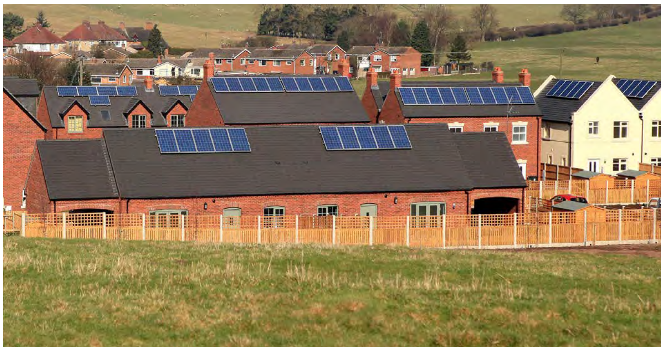
This new development in Himley Lane, Swindon, references typical barn forms within the scheme by including long, narrow buildings with pitched roofs. These building types are at the edges of the development, creating a sensitive edge with the adjacent landscape and a recognisable pattern in building heights which become lower towards the edges.
