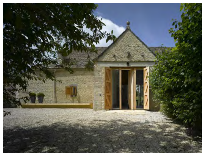
This barn conversion has retained old elements whilst adopting a contemporary style. Retaining the old walls provides character and is a reminder of its past farming history. The historic natural stone sits comfortably alongside more modern materials.
