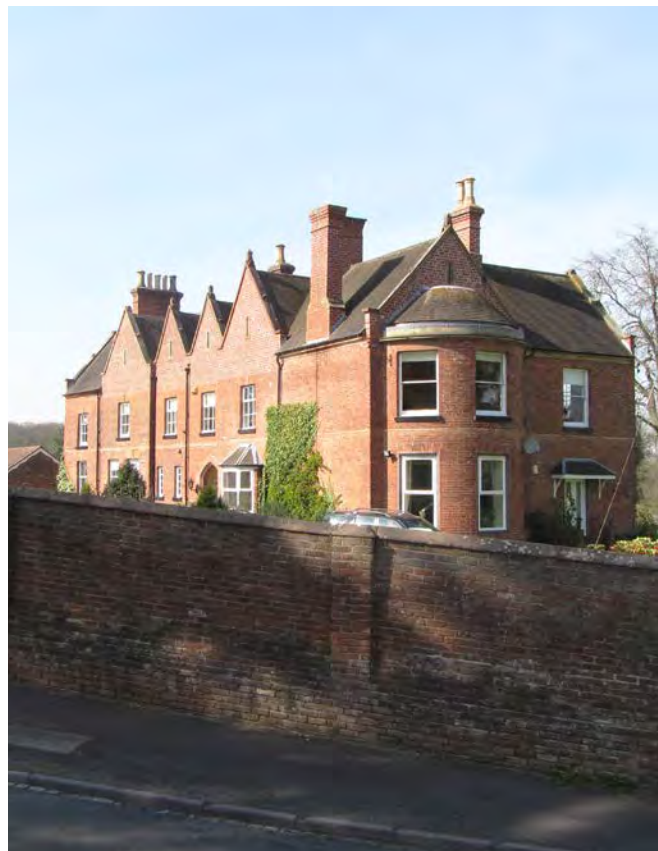
Enville Manor is typical example of historic building in South Staffordshire, with red brick, clay roof tiles and timber framed windows. New development should respect and respond to these historic design features.
