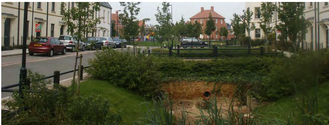
This artificial swale and channel has been designed to manage surface water run-off and provides an attractive and functional addition to the street.
