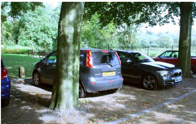
This parking in Kinver has been sensitively designed around mature trees with permeable surfacing to minimise damage to the existing retained trees.
