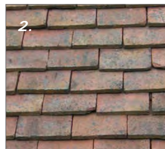
2. The most common roofing material is the red-brown clay tiles made from local Keuper Marl Clay. The clay tiles - called plain tiles - are of small scale, typically 265mm x 165mm, with a fine sand texture.
