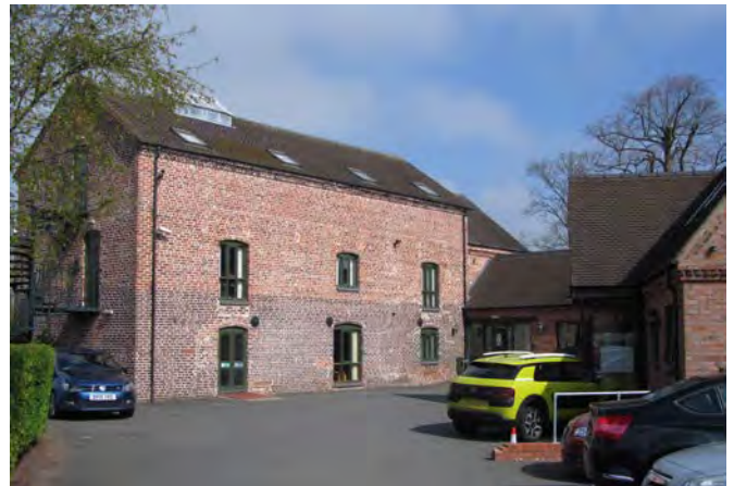
An example of a refurbished mill in Penkrige. Important qualities which have been retained include the simple building form and brickwork detailing.
