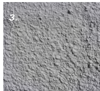
3. Rendered surfaces on the District's historic buildings were painted in a limewash, limited to a range of colours including cream, near white or stone. Brighter and pastel colours are not widely found.
