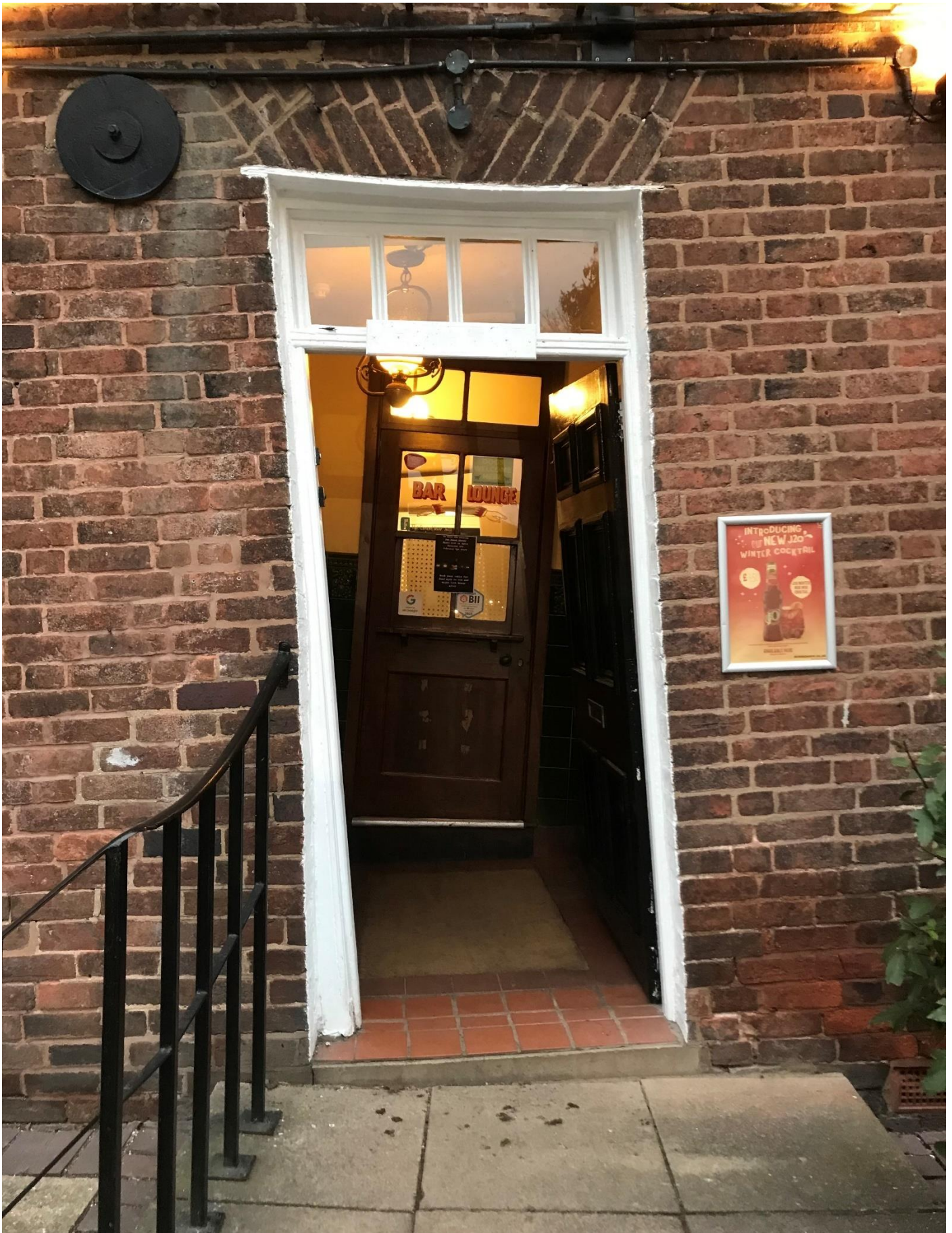
Photograph of front door. Not exterior door, and interior door with sash for servery. Modern step and handrail to left. (Ed Higgins, January 2023).
