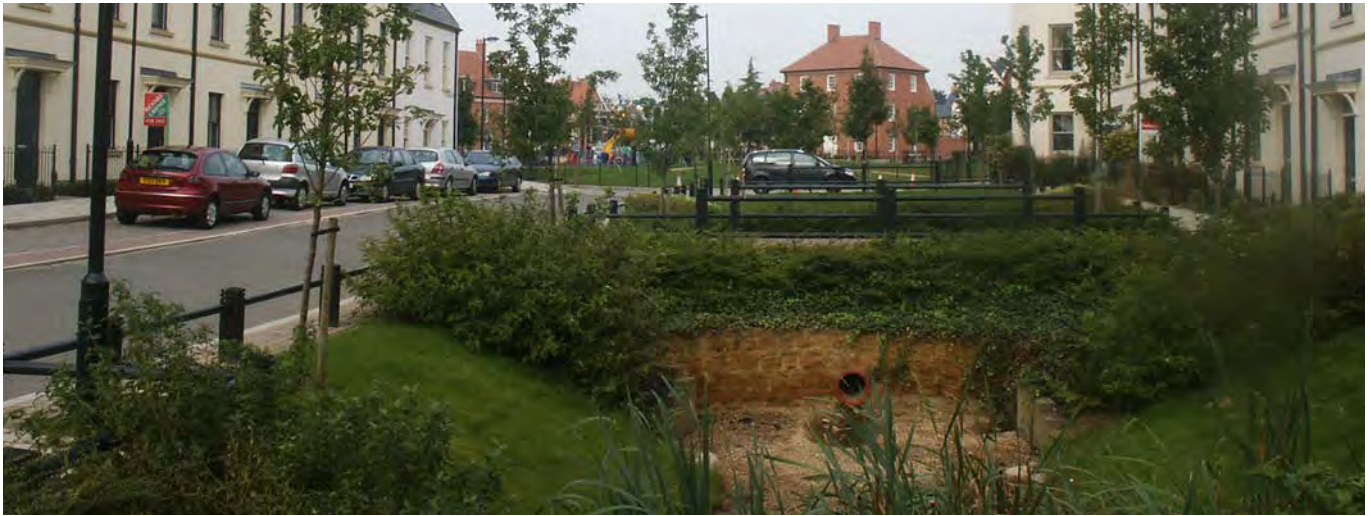
This artificial swale and channel has been designed to manage surface water run-off and provides an attractive and functional addition to the street.
